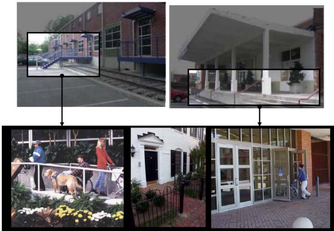
Figure A1. Examples of buildings, illustrating “visual character” in the BeltLine development guideline, have inaccessible entrances (top photographs). Special attention needs to be paid to front entrances usable by all ability and age levels (bottom photographs).
